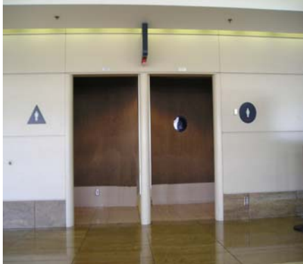
EXISTING VESTIBULE CONDITION AT A LAX TERMINAL 5 RESTROOM
