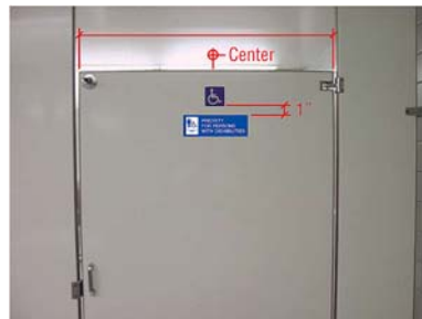
Typical location of decal installation.
