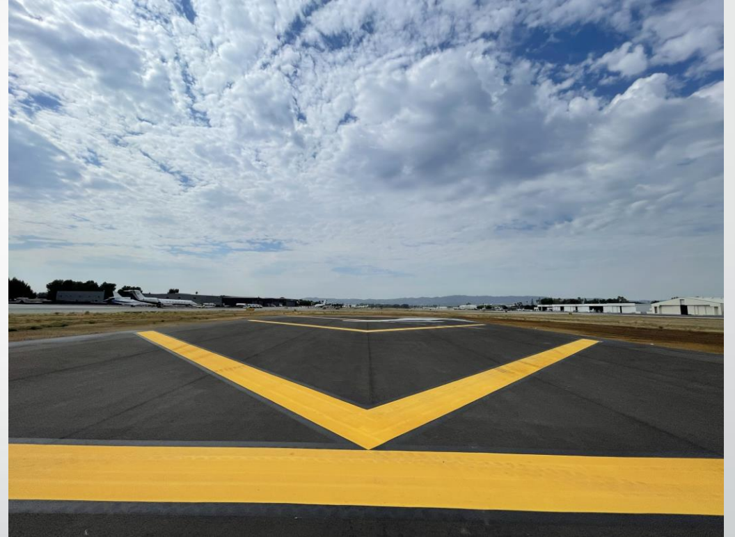
New southern blast pad on 34R
