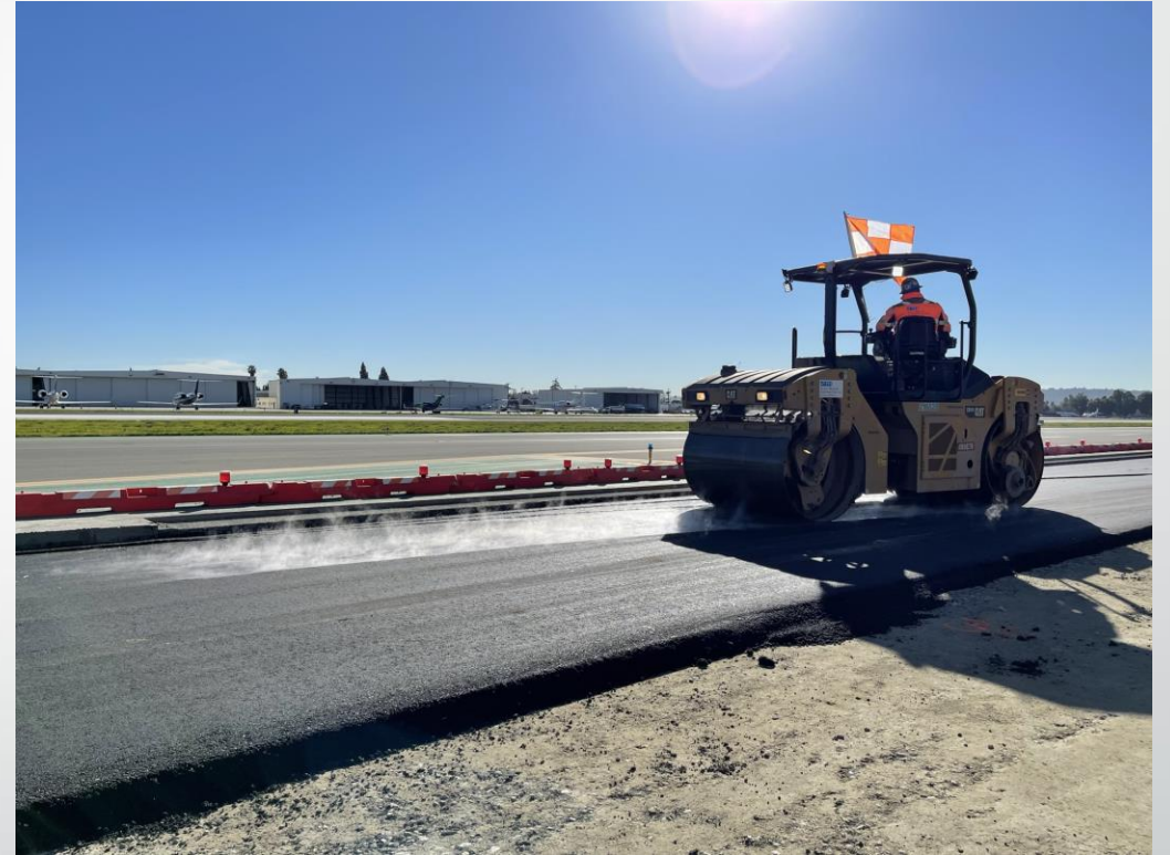
Asphalt paving on Runway 16L
