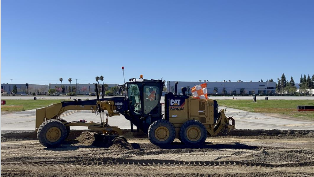
Grading operations on 16L
