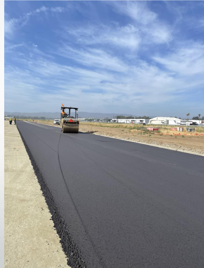
Asphalt paving on Runway 16L
