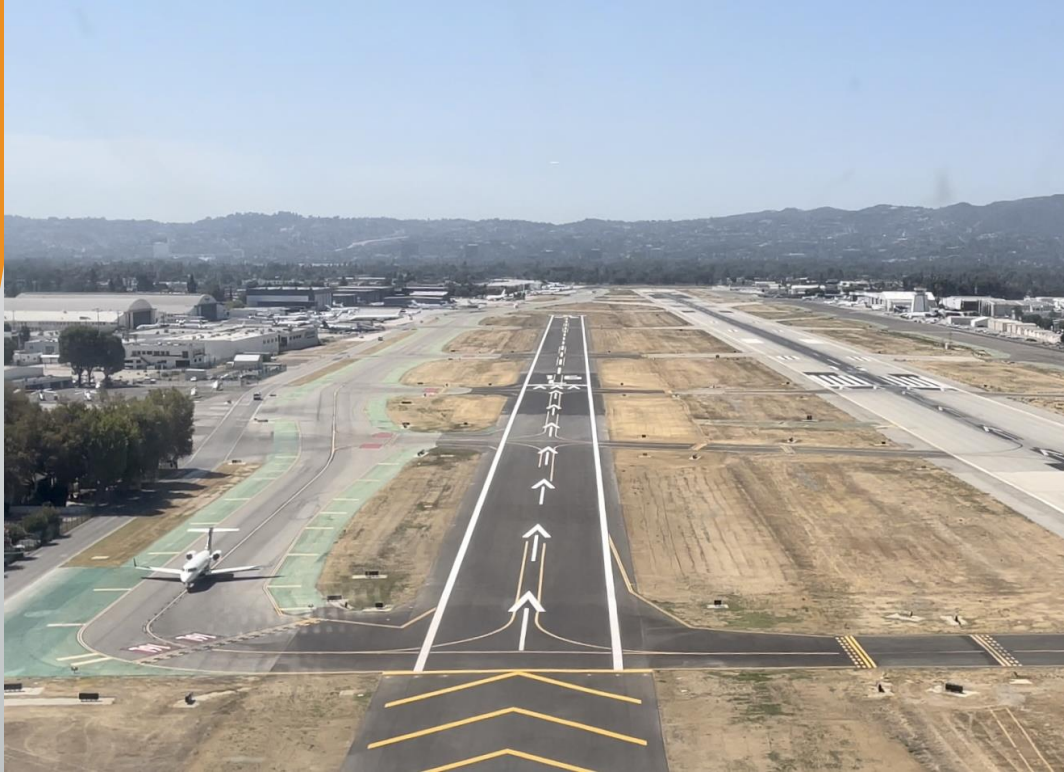
Approach to recently completed 16L
