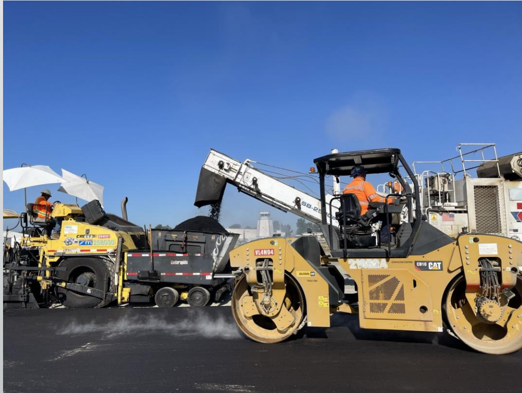
Asphalt paving on Runway 16L
