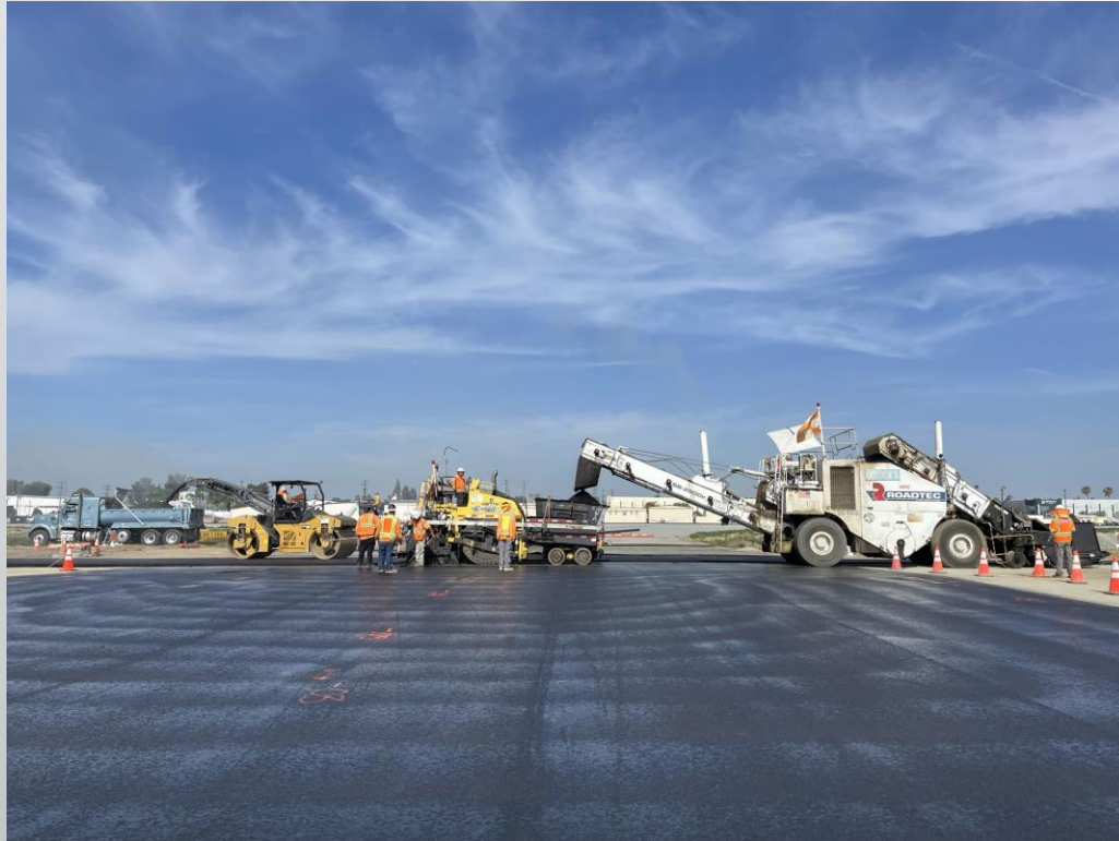
Asphalt paving on Runway 16L
